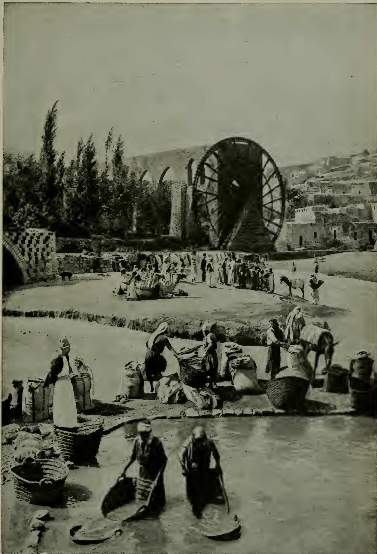
This huge water-wheel at Hamah, in northern Syria, 75 feet in diameter, is the largest in the world. The wheel runs without stopping day and night all the year round, and is used to raise water in buckets to the arched stone aqueduct for irrigation purposes. In ancient times the town was called Hamath, and was the capital of a Syrian kingdom which the kingdom of Israel touched in the time of Solomon.
